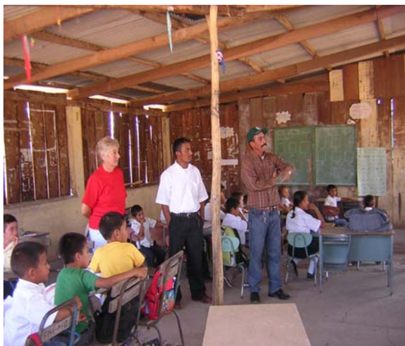
Large school, before repairs
