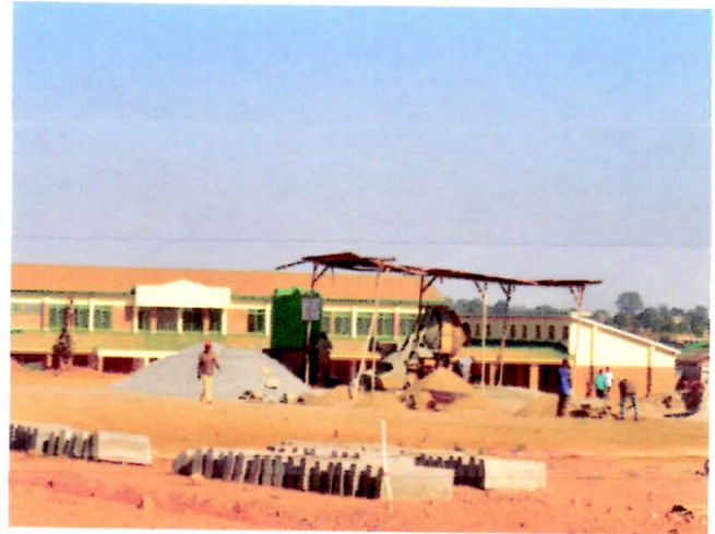
Construction workers keeping very busy as opening date approaches!
