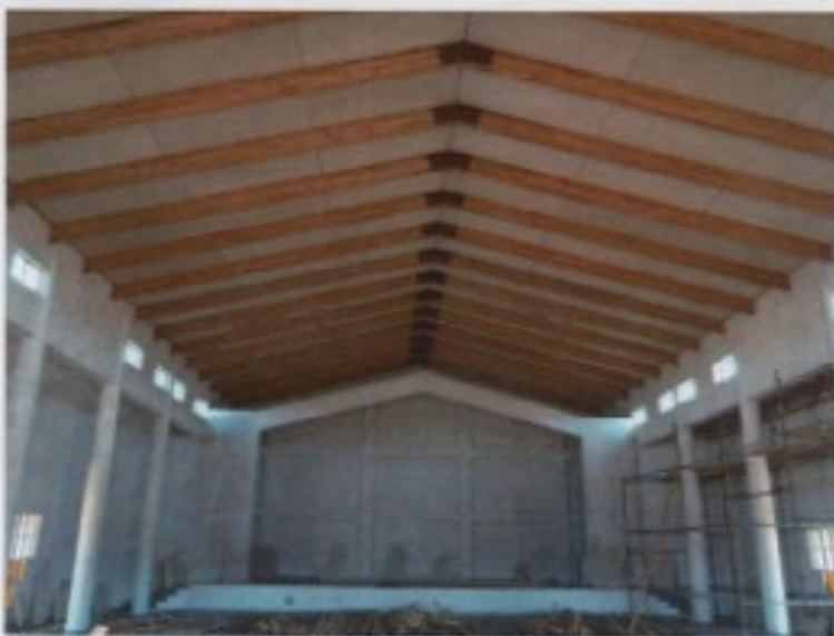
Inside Conference Hall – almost finished!
