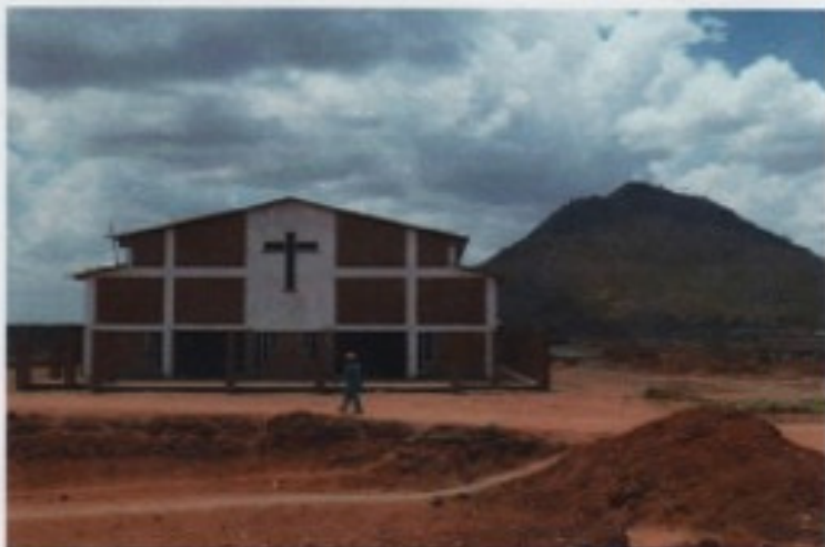
Conference Hall – centre of future activities
